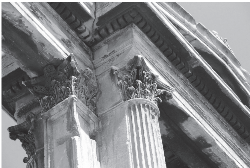
Figure 15.3 Traces of orange-brown paint on the attic of Hadrian's Arch.
