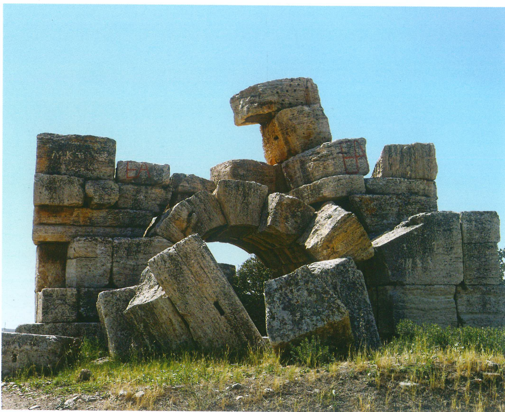
The ruins of the water distribution terminal.
