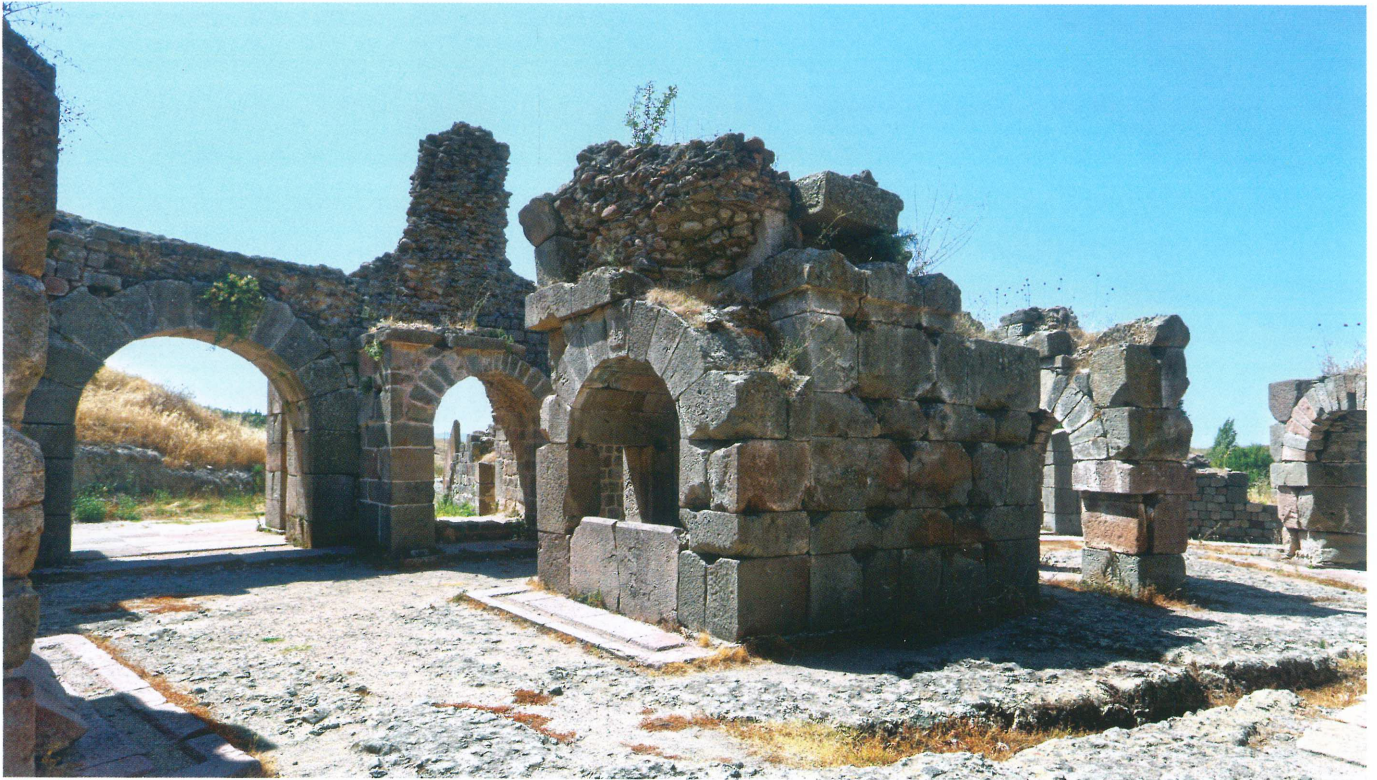
The treatment building.
