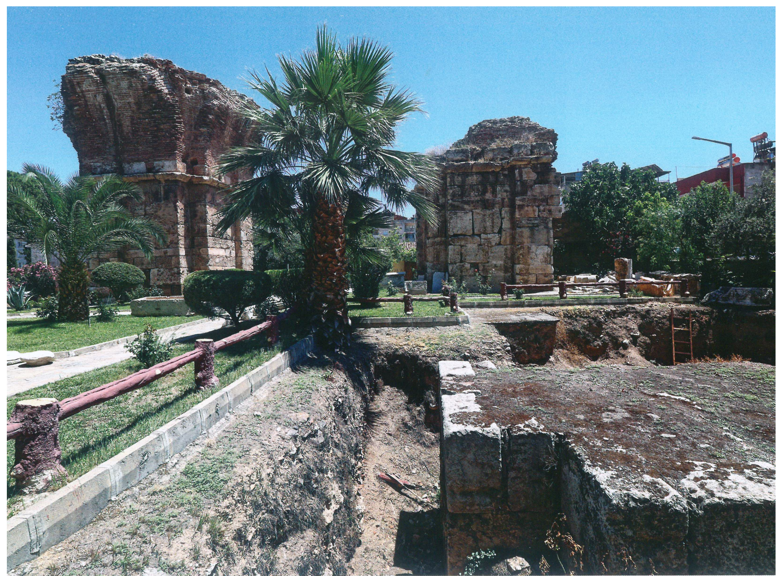
The foundations of the church.
