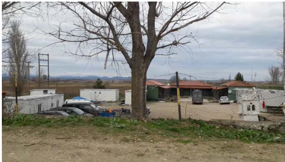
Figure 4: Video Still of the Poros facility (source: LK)
