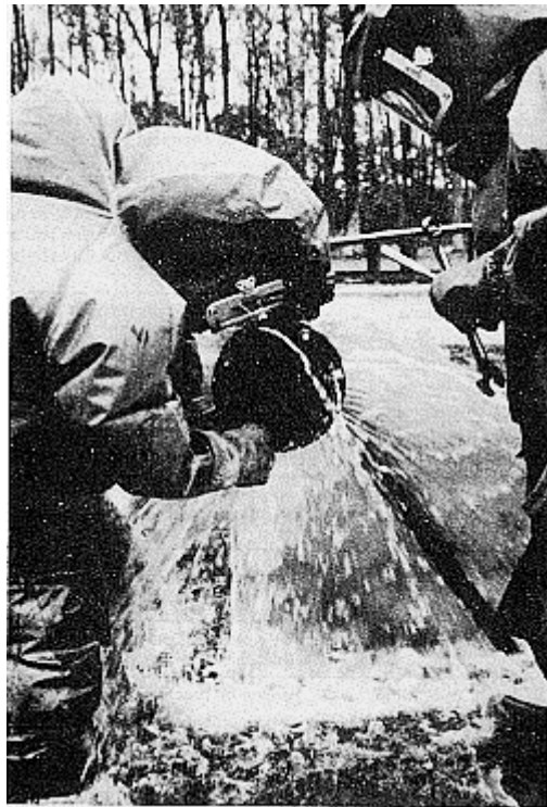
The training program should involve field drills that simulate emergency situations. Here workers wearing Level A personal protective equipment repair a leaking pipe as part of a training exercise.
