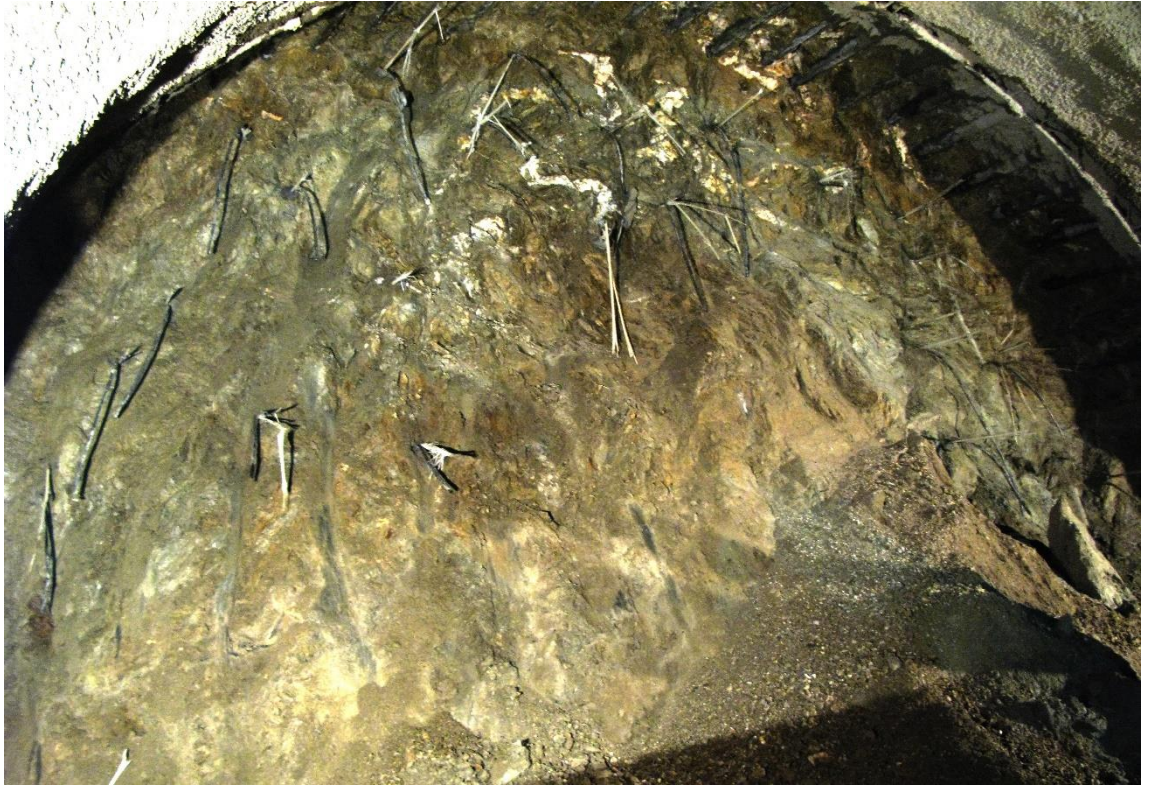
A.15 Slightly weathered metasandstone. Station tunnel (~ 18 m dia.) excavation face, side drift – Line 2, “Peristeri” station.
