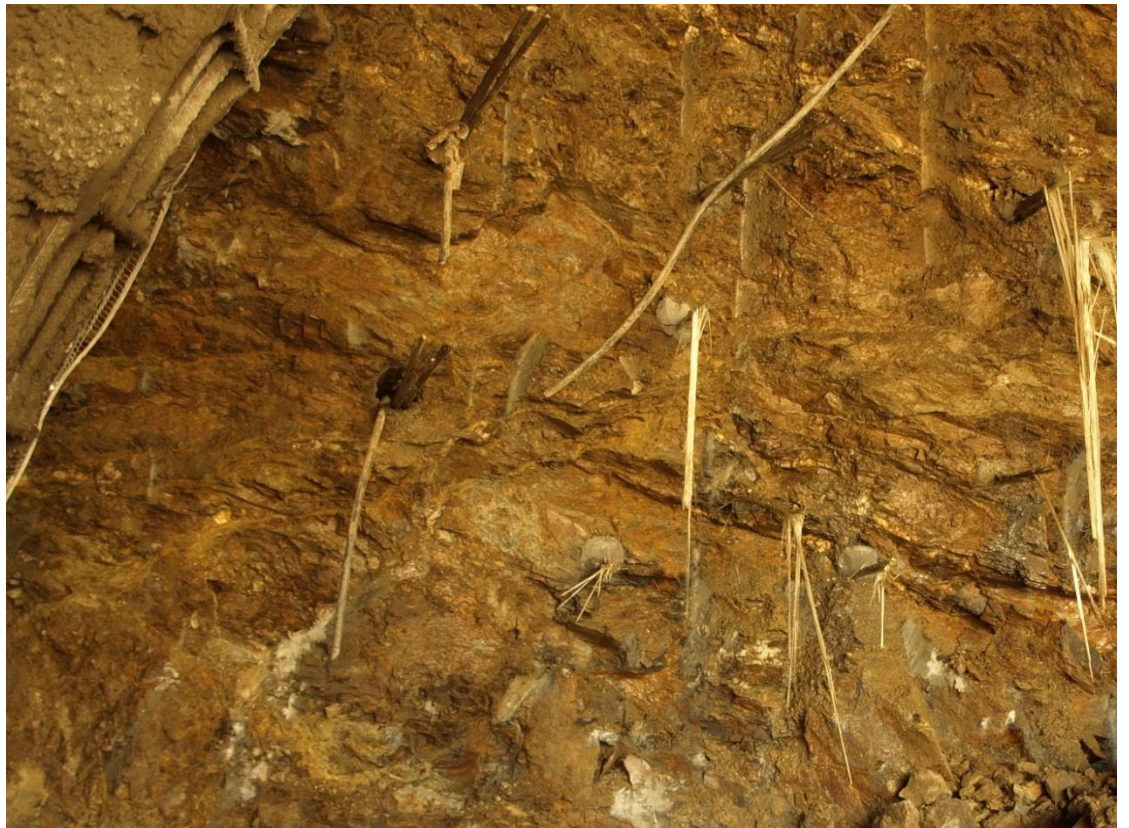
A.15 Slightly weathered metasandstone. Station tunnel (~ 18 m dia.) excavation face, side drift – Line 2, “Peristeri” station.
