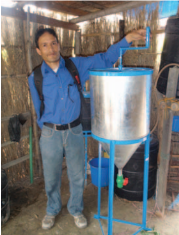
FIGURE 2 Pilot-scale installation in Nepal for the recovery of struvite from urine. Struvite was precipitated by the addition of bittern, a waste product from salt manufacturing, as a source of magnesium. After 10 minutes of mixing and 24 hours of settling, struvite was collected on a screen at the bottom of the reactor. SOURCE: TILLEY ET AL. 2009A; USED BY PERMISSION FROM EAWAG
