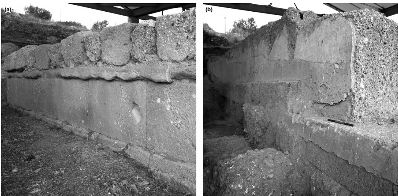
FIGURE 4.4 Detail of the south wall socle of (a) Building E and (b) Building D PHOTOS BY AUTHOR; COURTESY ÖAW/ÖAI ATHEN
