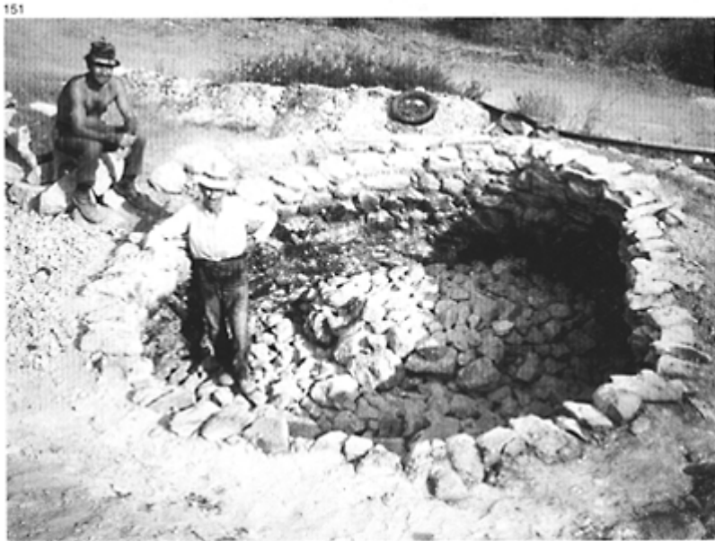
151 Completion of the loading of the kiln in fig. 149.
