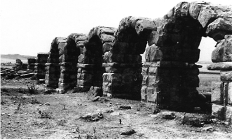
562 The massive arcaded section made of rusticated stone blocks of the aqueduct of Mactaris (Maktar) in Tunisia. Here a projecting cornice was used to support the centring.
