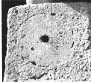
124 Four spike holes around the edge intended for the fine positioning of the shaft of a column. Forum of Pompeii.
