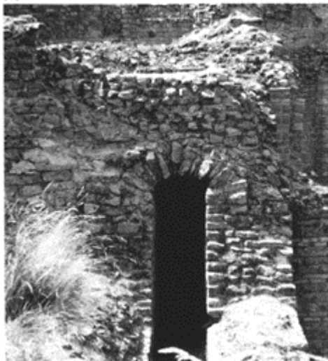
618 A tunnel separating the retaining wall, left , from the wall of the building, right , at the cryptoporticus of Bavay (Nord).
