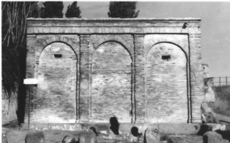
577 The castellum aquae of Pompeii near the Vesuvius Gate, the highest point of the city.
