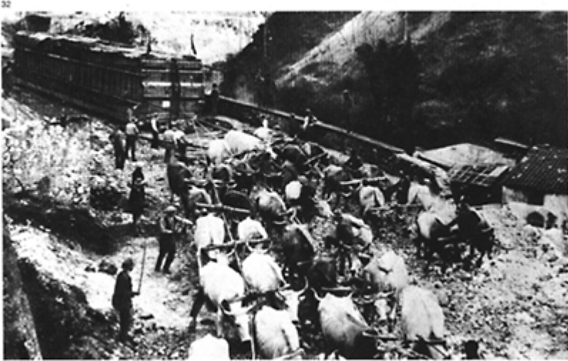
32 Mussolini's monolith being transported on a sledge, pulled by a team of sixty oxen, Carrara, 1928. (Photo: Hrand.)
