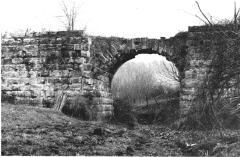
658 The Ponte Amato, on the via Praenestina , below Gallicano. On each side of this single-arched bridge is a large stone mass to avoid a fall in the level of the roadway.
