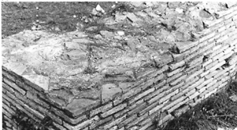
348 Masonry wall faced with triangular bricks. Ostia, beginning of the second century.
