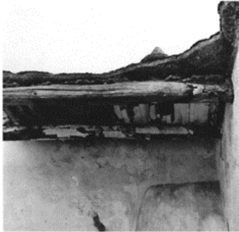
469 Ceiling of a ruined farm at Pompeii, showing the same structure as ancient ceilings: the beams support a parquet on which a layer of mortar is placed.
