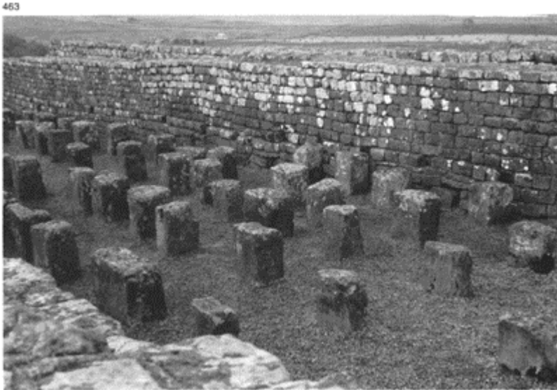
463 Hadrian's Wall: horrea of the garrison of Borovicus (Housesteads). Sockets and small supporting columns for the floor joists.
