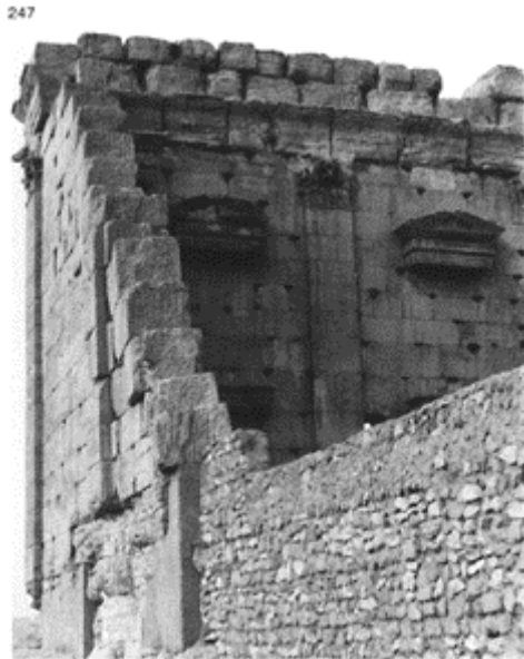
247 Wall made up exclusively of bonding blocks: peribolos of the Temple of Bel at Palmyra; first century
