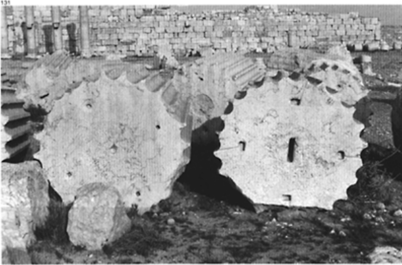
131 Column drums from the Temple of Bel, Palmyra. The drum on the right (upper face visible as shown by the lewis hole) supported that on the left. The sockets of the dowels are wide to allow for the lead sealing. On the lower surface of the other drum the holes for inserting the dowels dry-jointed are narrower. Note the slight depression of the centre.
