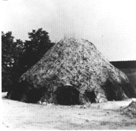
152 Exterior cone, or lamia , of the kiln at Foca, during the burning. The air-vents, or eyes, open at ground level.
