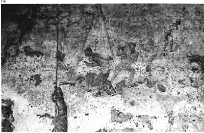
118 Painting from the House of Siricus showing a scene on a building site. Pompeii, VIII, 5, 26–57.
