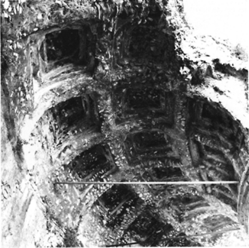
435 An angular vault of concrete masonry moulded on a centring in which the outline of the coffers had been prepared. Temple of Fortune at Praeneste. End of the second century BC.
