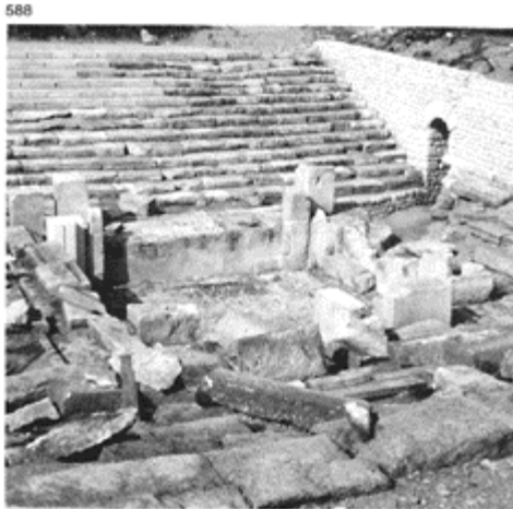
588 The monumental fountain at Argentomagus (St-Marcel, Indre). The four pillars in the basin supported a roof. The supply, at least in its final state, arrived via a wooden pipe under the steps.
