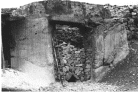
148 Lime-kiln on the road to Epidaurus (Peloponnese) in the course of being loaded.
