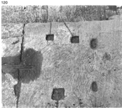
120 The top bed of a block from the foundations of the Roman Temple of Euromos (Caria). Note here, from left to right, the sealing clamp, three sockets for vertical dowels (with channels for the overflow) and two spike holes, thus enabling the block to be clamped to the joint of the upper block.
