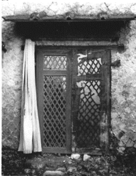
676 A door with double lattice leaves at Herculaneum (Eastern Insula II). The left-hand door is modern.
