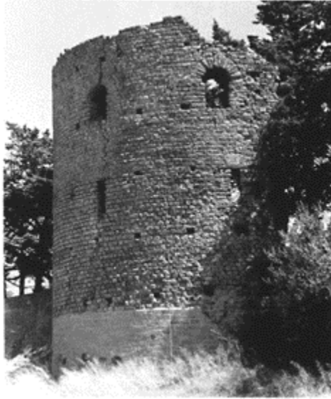
320 A tower in the walls of Fréjus faced with opus vittatum in which the putlog-holes are visible. Beginning of the first century AD.
