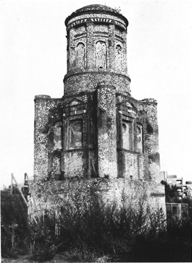
299 La Conocchia (the Distaff), the funerary monument erected on the via Appia near Santa Maria Capua Vetere. A late example of masonry faced with opus incertum , erected at the end of the first century or the beginning of the second. Notice the use of brick for
