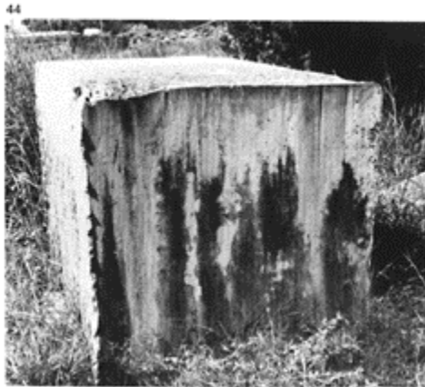
44 A sawn block of marble on the building site for the Temple of Venus at Pompeii.
