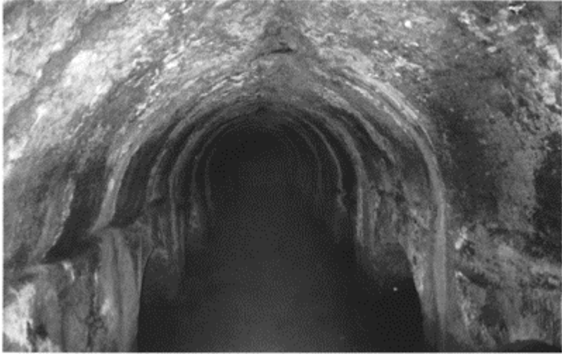
576 One of the five chambers of the large cistern of Albano, called 'il Cisternone', built in the Severan period and still in service today supplying the town. Capacity: 10,132\text{m}^3 .
