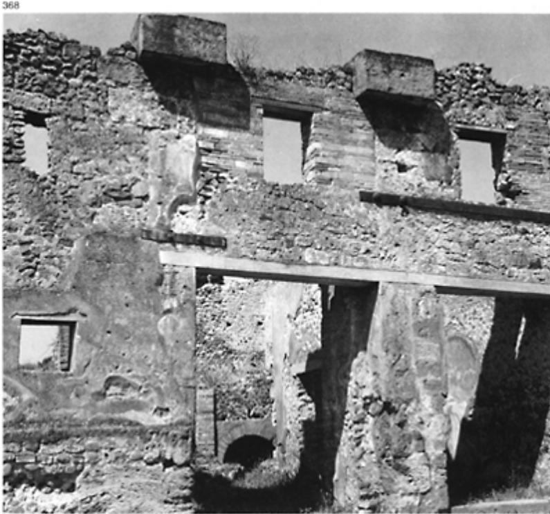
368 Pompeii, façade of a domus turned into a bakery after the earthquake of 62. The high door framed with cubic capitals was hidden by the addition of a first floor; the oven, visible at the back, was constructed in the atrium (VIII, 4, 26).
