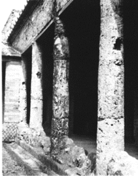
267 Villa of the Mysteries at Pompeii, colonnade made of Sarno limestone, initially belonging to the Samnite period.
