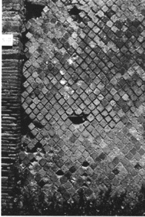
188 Wall of reticulate construction, in which can be seen the putlog holes of two levels of scaffolding, each with a small lintel. Pompeii VIII, 2, 30; c. 70.
