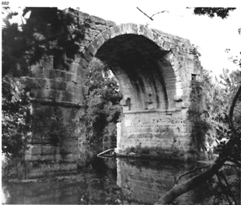
662 The surviving arch of the beautiful bridge of Ambrussum crossing the Vidourle. On the sides of the arch the
