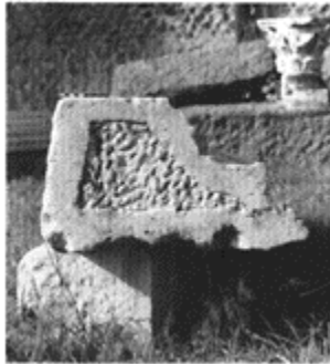
112 Anathyrosis rebating (or bevelling); only the edges of the frame are in contact, on this snugly fitting joining surface of a cornice element. Temple of Venus, Pompeii.
