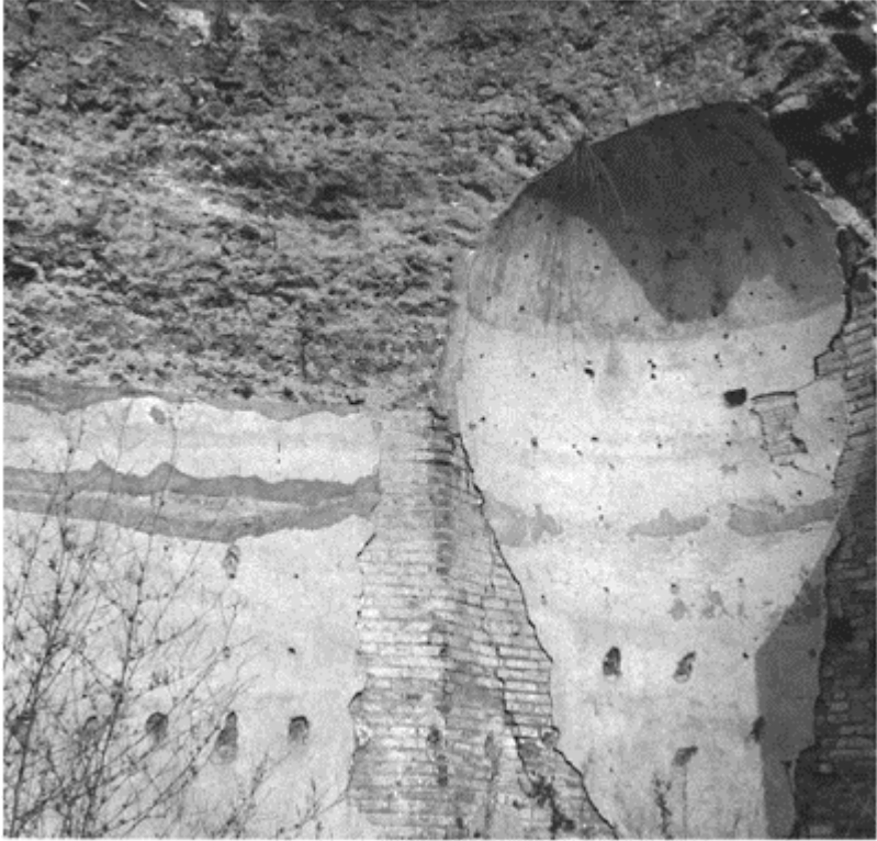
442 A dome with niches in the laconicum of the Central Baths at Pompeii. Notice here three successive layers of material: bricks for the drum, opus caementicium , tufa rubble for the haunches and thin honeycomb lava for the capping. Between 62 and 79.
