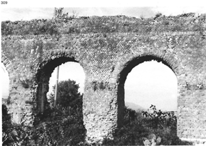
309 Aqueduct of Minturno ( Minturnae ). Masonry bonded with lime mortar with reticulate facings, the quoins and arch crowns made of small blocks. Augustan period.
