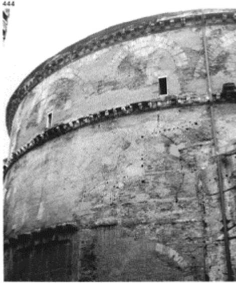
444 The Pantheon (118–25), a network of stiffening arches reinforcing the masonry of the drum.
