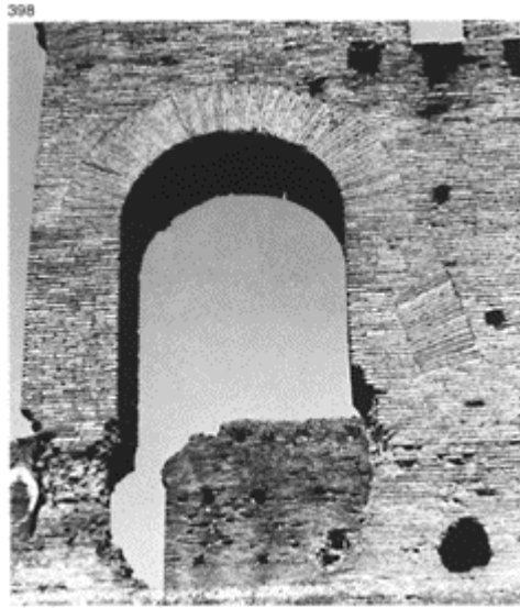
398 An abutted buttress built into the wall mass and following the actual direction of the forces. Villa of the Quintilii; c. 150.
