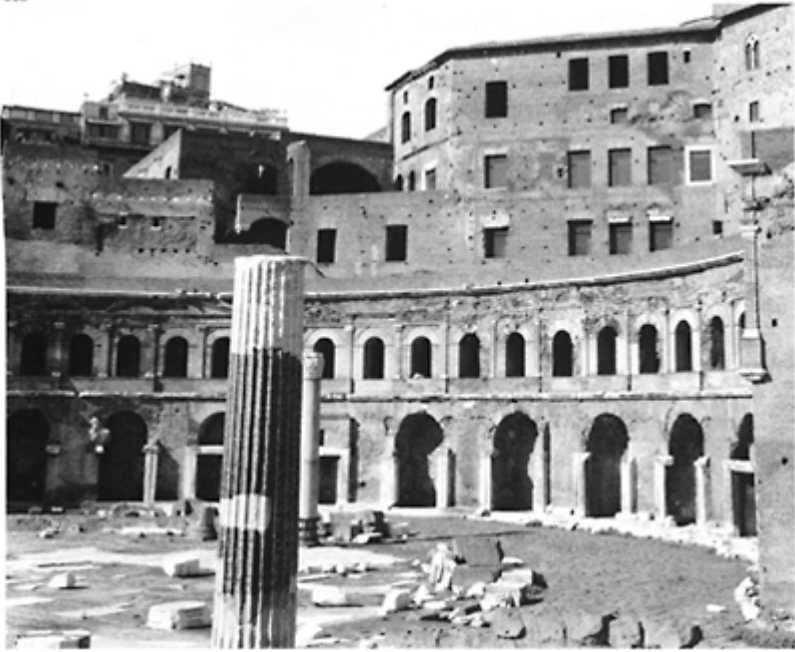
352 The exedra of the Markets of Trajan: a systematic use of brick facings with frames, bases and capitals of travertine; presumably this dual coloration was intended to remain visible.
