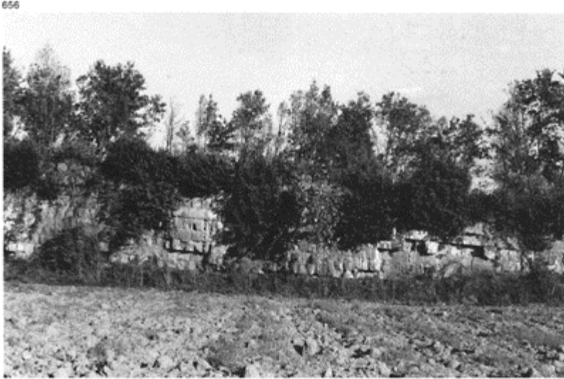
656 An embankment on the via Flaminia , approaching a hill near Civita Castellana, known as the 'Muro del Peccato'. The work on this began in 220BC. This large construction, similar to the viaduct of Valle Ariccia, indicates a preference for a straight course rather than bends, which allow a gentler incline, because of the appreciable shortening of the distance covered.
