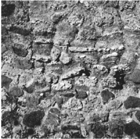
366 Pompeii, restoration of a wall after the earthquake of 62. Among the reused material are pieces of opus signinum paving (VI, 7, 2).
