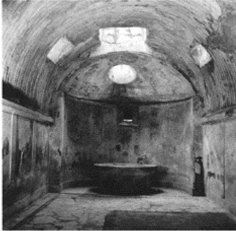
640 Stuccoed vault with light well in the caldarium of the men's baths in the Forum Baths at Pompeii.
