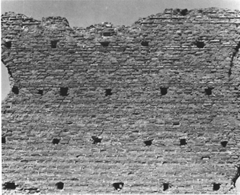
184 Transverse putlog holes in the aqueduct of the ville dei Sette Bassi ( via Latina ; c. 140)
