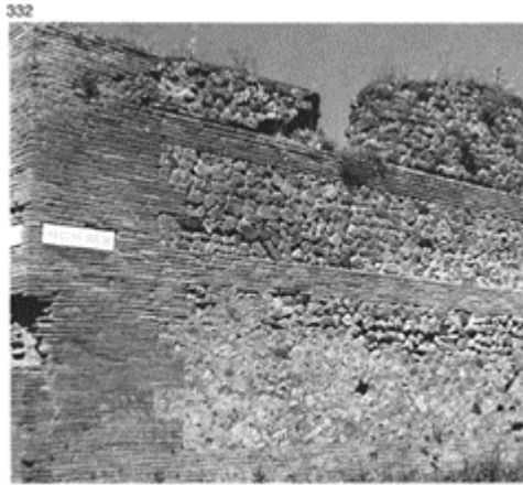
332 Opus mixtum from the last phase at Pompeii (62–79) made up of opus incertum with courses and quoins of brick (VI, 10, 15).
