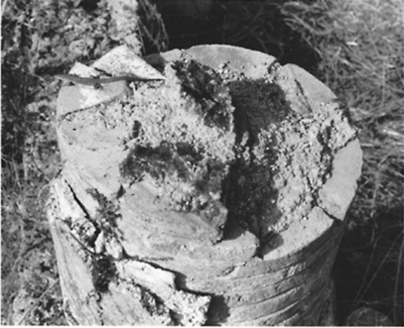
371 Column shaft made of bricks in irregular quarters; diameter without the rendering: 45cm. House of Terentius Proculus at Pompeii.
