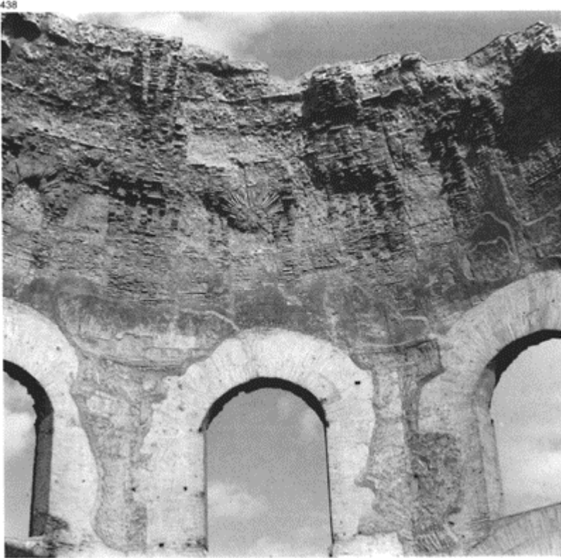
438 The interior of the dome of the 'Temple of Minerva Medica' in Rome. The transition from a tensiled to a circular shape is carried out by means of a progressive and undetectable tapering of the masonry. The structure is that of coffered and ribbed masonry, defined by brick frameworks containing a fill of rubble. Notice that the strong ribs radiating out distribute the pressures
