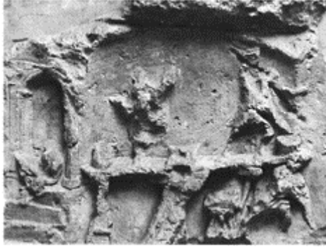
178 Relief from the Musée de Sens, showing masons and a painter applying a rendering using trestle scaffolding. (Length: 101cm; height: 85cm.)
