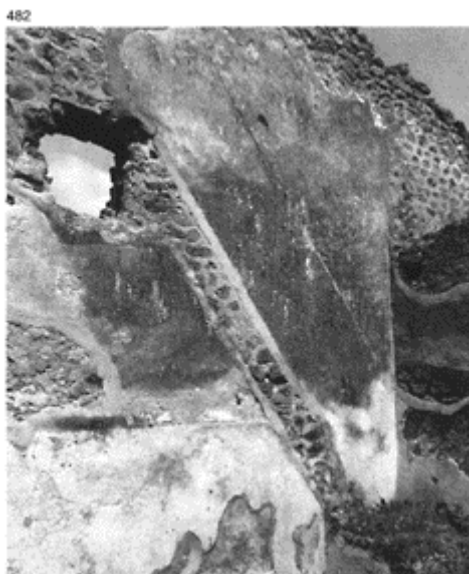
482 The remains of a wooden staircase support with a masonry base. The decoration of the rendering followed the incline as far as the upper landing. Pompeii, IX, 1, 4.
