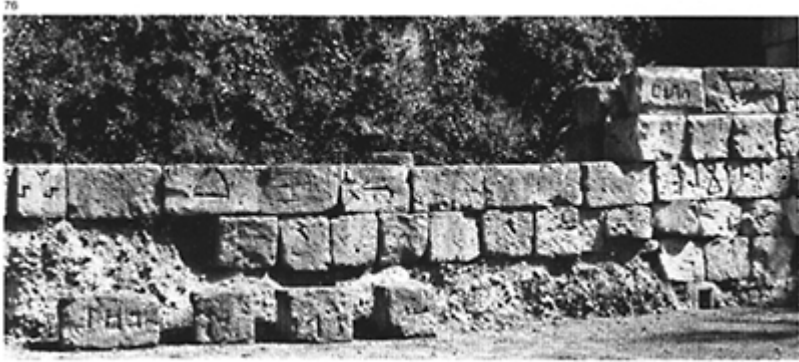
76 In the Republican period, the stone-masons, following a Greek custom, placed their mark on the blocks. Walls of Bolsena, third century BC. This custom was to reappear occasionally in the Imperial period, notably in North Africa.
