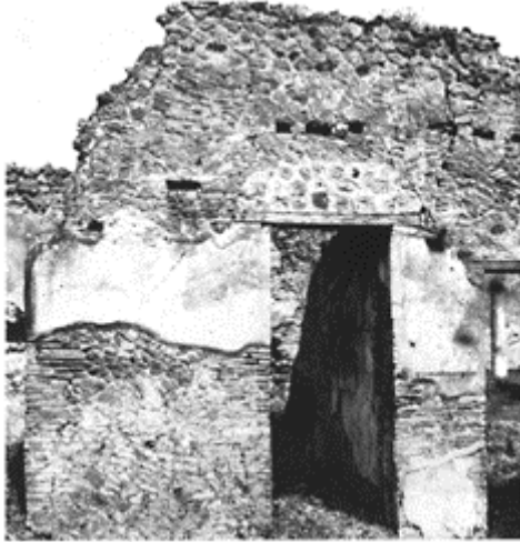
365 Pompeii, reconstruction after the earthquake of 62. Wall made up of varied terracotta material: bricks, tiles, fragments of amphorae (IX, 6, 3).
