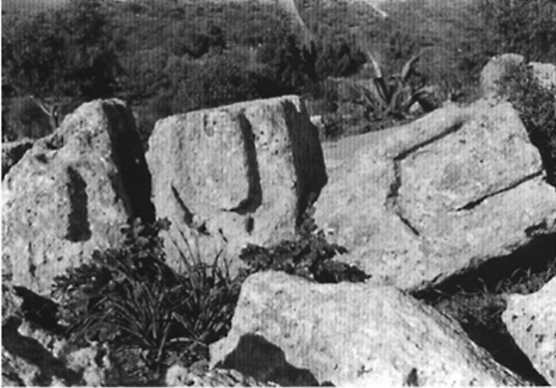
101 Side grooves on blocks from the Greek temple in honour of Juno Lacinia at Agrigentum (fifth century BC). The Romans never adopted this system of lifting though it was known in Sicily.
