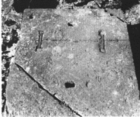
129 Pi clamps, of which only the vertical pieces are sealed with lead. Forum of Bavay.
