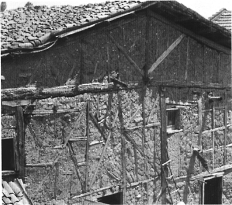
134 Timber framing with clay infilling in the traditional architecture of the region of Bursa (Turkey).
