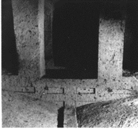
485 Etruscan tomb at Cerveteri showing the ridge beam supporting the two slopes of the roof and, on the tympanum, the jointing of the pieces forming timber framing on the façade; c. 500 BC.
