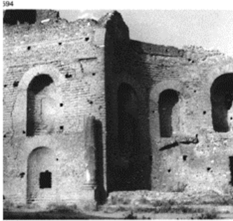
594 The large nymphaeum of the villa of the Quintilii, on the via Appia between Rome and Bovillae, built in the third century AD. The large apse containing the basin was covered over with a half-dome. The right-hand part of the structure is concealed by a medieval construction; a special aqueduct, as at the Villa dei Sette Bassi, supplied the building.
