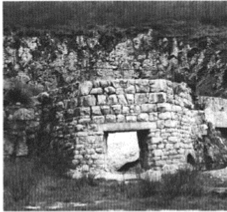
147 Lime-kiln situated right at the foot of the quarry supplying it at Itri, southern Latium.
