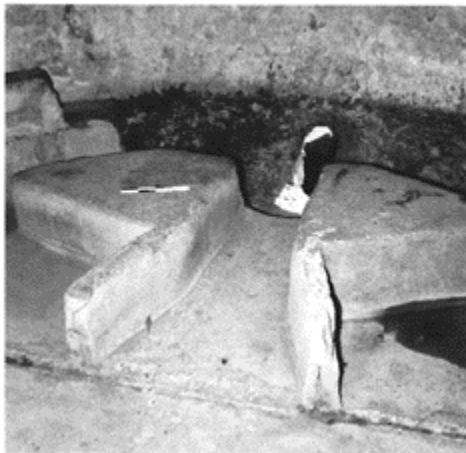
578 Division of the water into three channels in the castellum aquae at Pompeii. In front of the triple divider is the housing of the lead plate which once formed a dam for the water to
