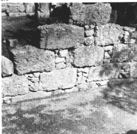
275 Bolsena, wall of 'chequer-work' construction at the 'domus with atrium' (beginning of the second century BC). The dimensions of the infilled sections are relatively small
