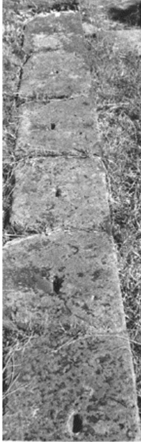
104 Lewis holes in the floor slabs of the threshold to a public building in Pompeii ('Tollhouse', IV, 1, 13).
