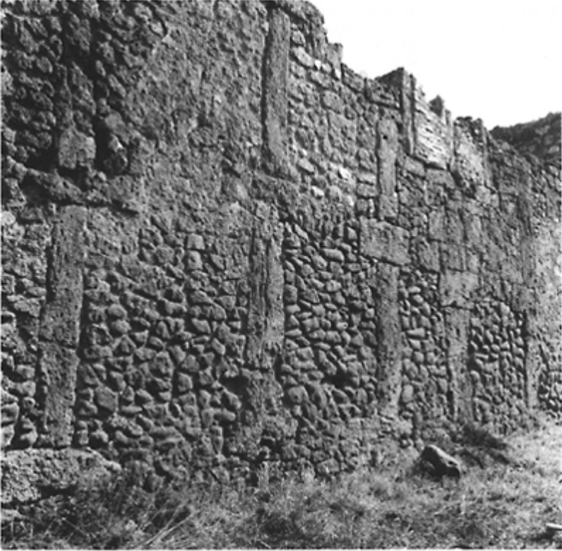
277 Wall of opus africanum with vertical chains of limestone blocks and infill of lava rubble. Pompeii I, 12, 1.
