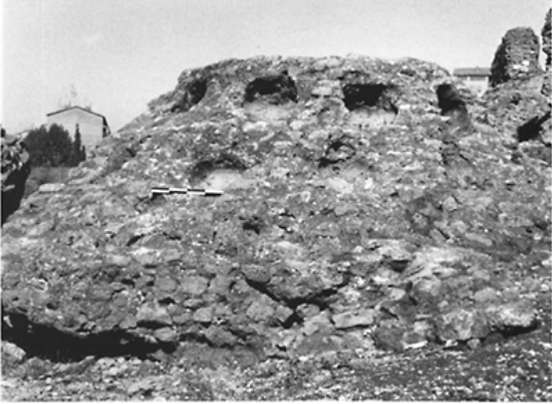
441 The capping of a dome made of tufa masonry, in which amphorae were sunk to lighten it. Large octagonal hall in the Baths of the Villa dei Gordiani, on the via Praenestina . Third century.
