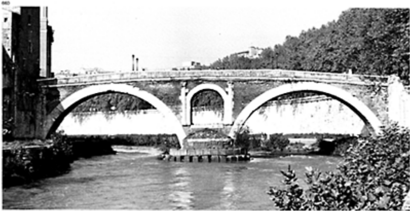
660 The Pons Fabricius built in 62BC to connect the Isola Tiberina to the Forum Boarium . The arch openings are 24.5m wide.
