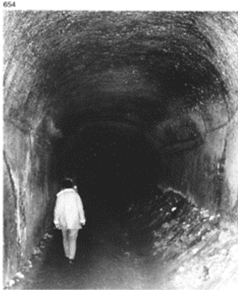
654 The 'grotto of the Sibyl'—a tunnel dug into the volcanic tufa in the Augustan period, between Lake Lucrino and Lake Averno. This allowed a rapid passage for pedestrians and vehicles between the facilities at these two stretches of water, themselves connected with each other and with the sea by an enormous canal, now filled in. Length of the tunnel:
