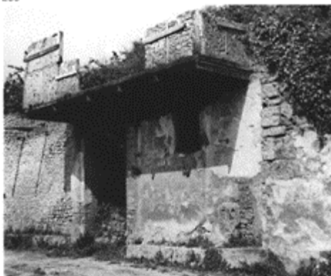
285 Timber-framed shutterings of a corbelled upper storey on the via dell' Abbondanza at Pompeii, III, 5, 2.
