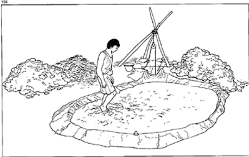
136 Mixing clay with straw as a defattening agent tempering by treading, in the preparation of puddled clay or unbaked bricks.
