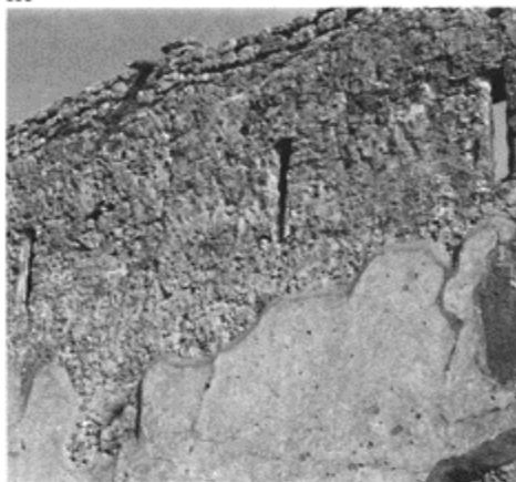
698 Slit openings on the ground floor of the House of the Faun; only the upper floors had large-size windows.
