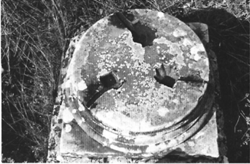
130 Socket holes of three vertical dowels in a column base. Imperial triclinium of Hadrian's Villa, 115 to 125.
