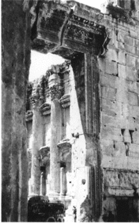
409 A lintel constructed of three elements, the Temple of Bacchus at Baalbek. Second century AD.
