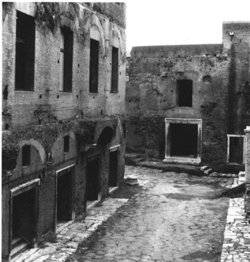
648 The via Biberatica in Rome, paved with lava, lined with pavements and shops, with commercial premises above, forming the Markets of Trajan.
