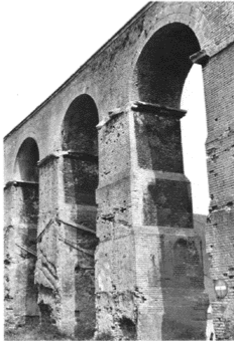
419 The arches of the aqueduct of Metz ( Divodurum ) at Jouy-aux-Arches, display a double row of voussoirs. The centrings for building
