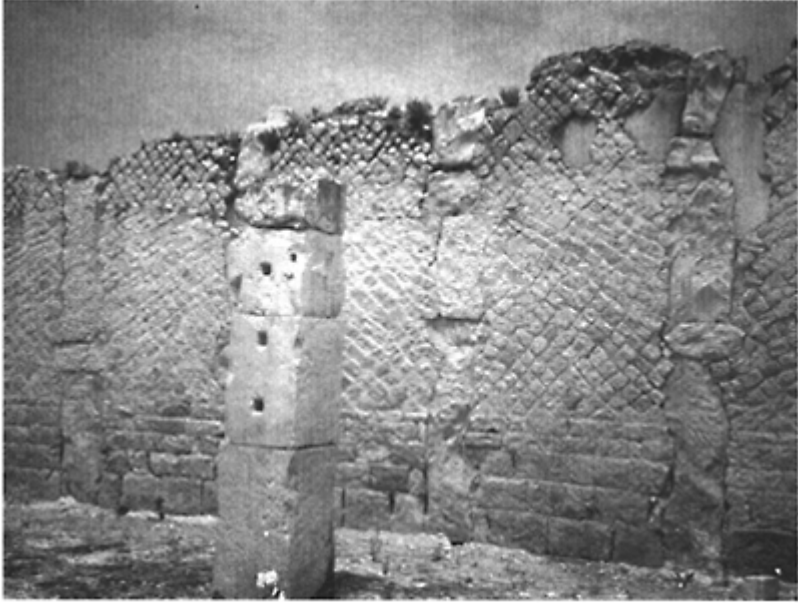
280 Building at Bulla Regia (Tunisia) with reticulated facings between vertical chains.
