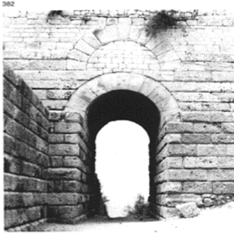
382 The Porta Rosa at Velia (Lucania) opened in a wall built c. 340BC. Width: 2.68m. Note the difference in the treatment of the blocks in the covering arch and in the relieving arch.
