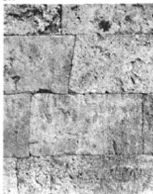
244 Walls of Pompeii. Second phase. Note the curvilinear joints from the cut of a saw.
