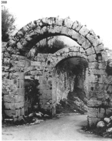
388 The Porta Maggiore at Ferentino ( Ferentinum ). The two arches of an opening 4.2m wide with a double row of short voussoirs are to be compared with the outflow of the Cloaca Maxima ; date around 80BC.
