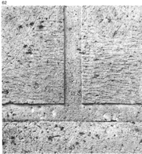
62 Rustication in part carried out with a stone-hammer, in part with a claw chisel, with the joints polished or
