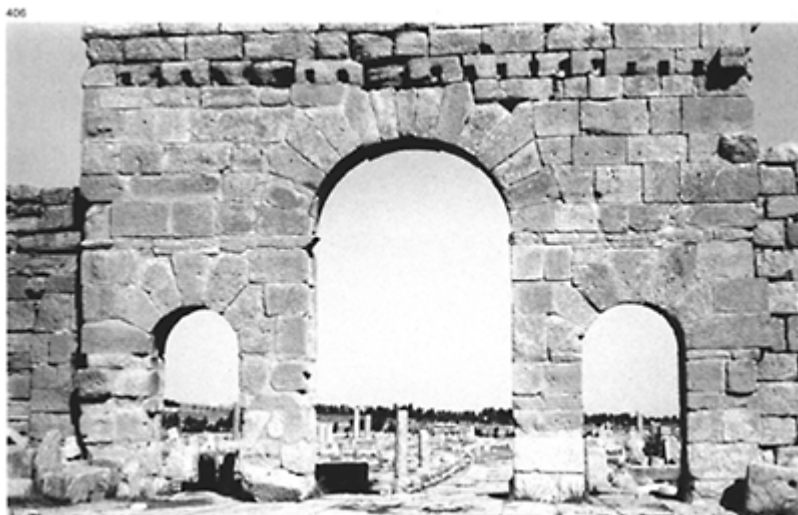
406 The Gate of Antoninus at Sbeïtla (Sufetula). The internal facing shows the random incorporation of the voussoirs in the construction of the wall.
