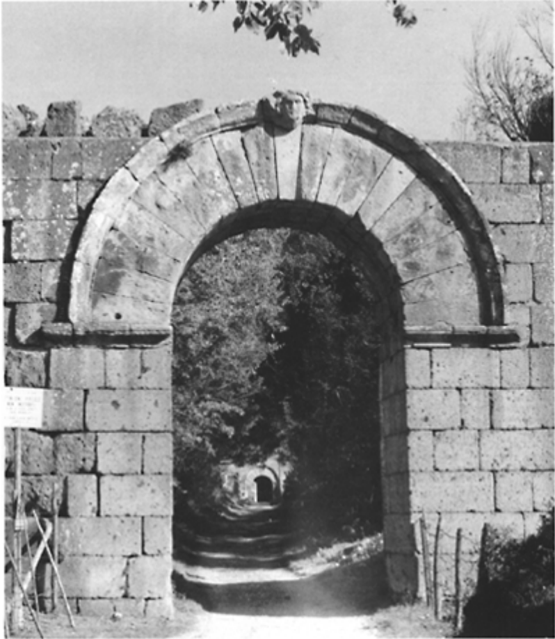
379 A true arch from the Gate of Jupiter at Falerii Novi dating after 241 BC. The long and narrow voussoirs have an archivolt added; it also has a very carefully made extrados. Width: 3.3m.
