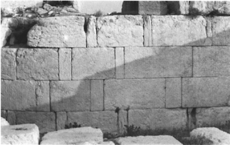
256 A systematic alternation of stretchers and headers is visible in the facing of Justinian's Wall at Palmyra; sixth century.
