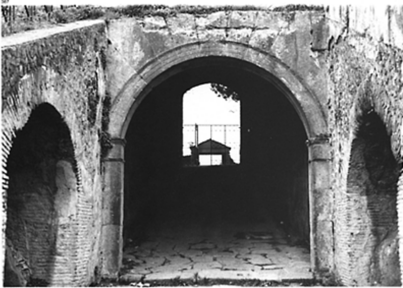
387 The entrance arch to the northern vomitorium of the amphitheatre of Pompeii with a span of 3.45m. The voussoirs are here incorporated into the rectangular shape of the passage; date around 80BC.
