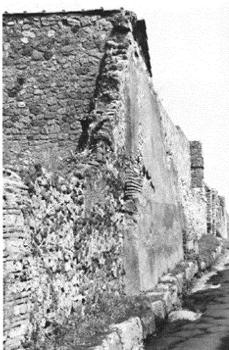
360 Pompeii, buttress-wall of brick and rubble stones, applied to a damaged building (Pompeii, VI, 2, 4).
