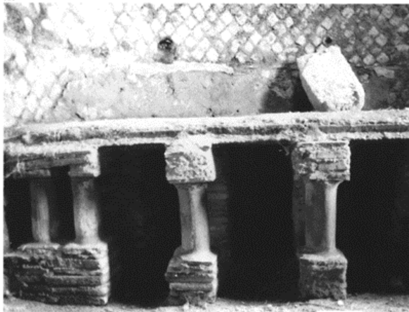
628 Hypocaust of a caldarium of the Baths of Baia (first century). The small columns were made up of terracotta elements, extended with bricks 20cm square. Height of the hypocaust cavity: 74cm; thickness of the floor: 14cm.
