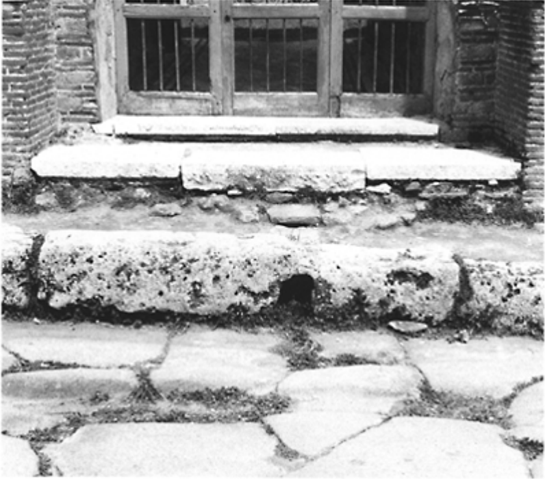
550 Outflow pipe of a cistern overflow in a domus at Pompeii. IX, 3, 5.
