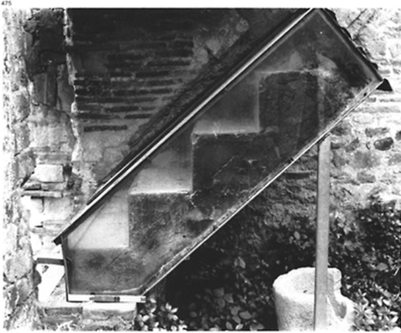
475 Detail of the wooden staircase in fig. 474, which had solid steps.
