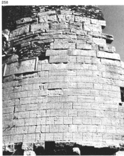
258 Facing of travertine on the tomb of Caecilia Metella. Because of the deterioration of the upper courses it is noticeable that the actual lengths of the blocks do not correspond to the regularly incised joints.
