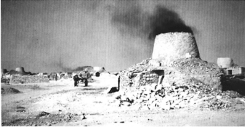
154 Mixed kiln in the region of Kairouan, with lime burning in the lower half and brick baking in the upper.
