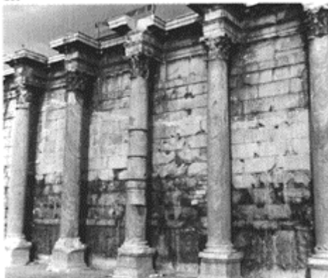
260 Fine regular marble construction, with drafted margins, resting on a row of orthostats; Library of Hadrian in Athens, c. 130.
