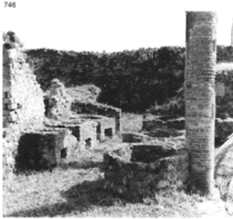
746 Furnaces and vats belonging to a dyer's installed in the peristyle of a domus after 62; Pompeii (VII, 2, 11).
