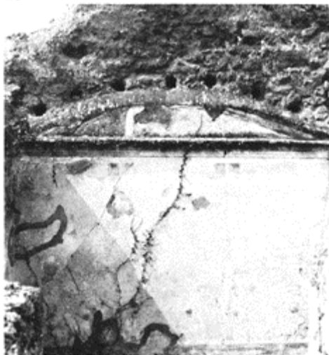
473 Remains of the sockets of the beams supporting a hanging vault, covering a room at Pompeii, IX, 5, 21.
