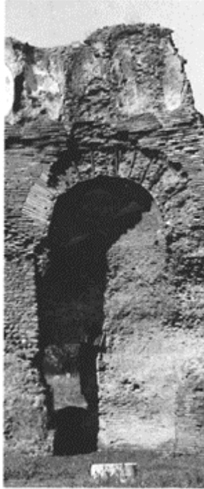
440 The apse of a large room in the Villa dei Gordiani, crudely covered by a semi-dome in an umbrella shape with very pronounced ribbing. Third century.
