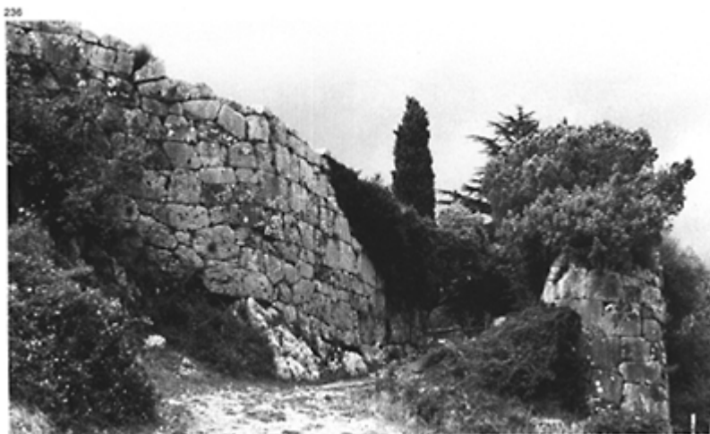
236 The Porta Maggiore of the acropolis of Norba (fifth to fourth century BC) with polygonal stone block construction of the third type. The foundation block of the left-hand corner is 3.05m long by 1.15m high and the same width; it weighs in the region of 10 tonnes. The gate opening is 6m wide.
