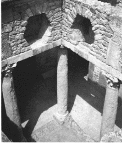
665 House of the Hunt at Bulla Regia , Tunisia. A sunken atrium with underground rooms for the hot periods. Fifth century.
