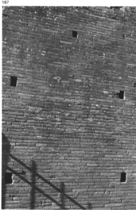
187 Putlog holes in a brick wall. Pompeii VII, 4, 24; c. 70.
