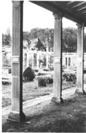
273 Rectangular marble pillars in the 'Hall of Doric Pillars' at Hadrian's Villa, 118 to 125. Only the corner pillar, with the square section, is of massive proportions.
