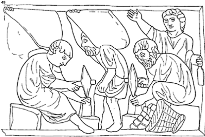
49 Stone-masons preparing stone blocks; their tool seen in profile could be a scabbling hammer (with two points) or a double-bladed stone-hammer. In the basket are the finished products. Relief from a tomb on the Isola Sacra, Ostia (drawn by JPA).
