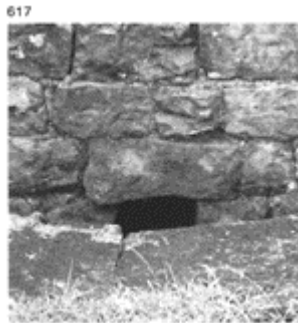
617 A drain for runoff water, Hadrian's Wall.
