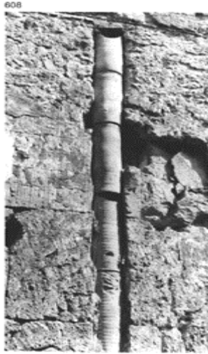
608 Drainpipes made of terracotta were protected by being sunk into a vertical groove so that they did not project from the wall. Pompeii, I, 3, 1.
