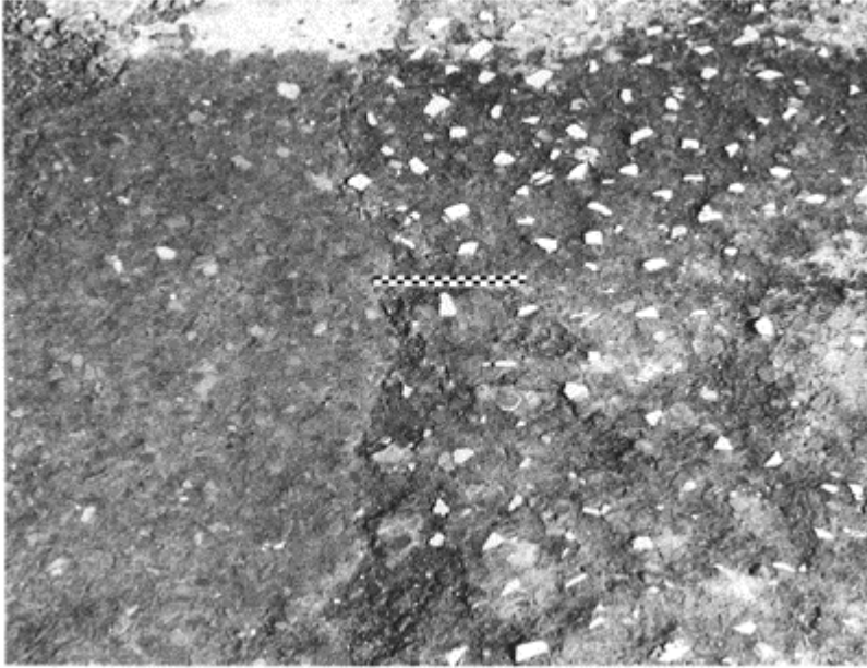
542 Pavement surface at Pompeii made of concrete with large ceramic fragments, dotted with white tessellae on the surface forming opus signinum (the Italian ‘coccio pesto’). Via di Porta Marina.
