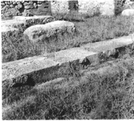
99 Lifting bosses, or tenons, on the slabs of stylobates at the portico of the Central Baths, Pompeii; they were being put into position at the time of the eruption of 79.
