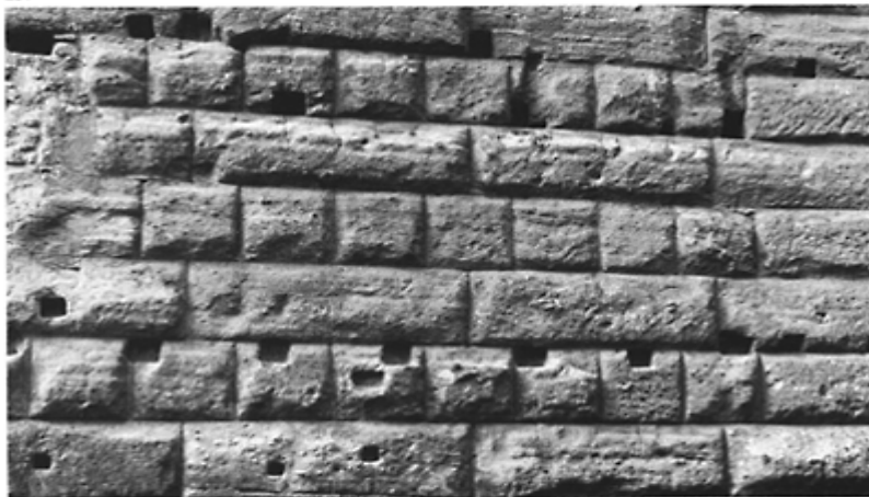
251 Detail of the wall of the Forum of Augustus showing the alternation of courses of stretchers and courses of headers.
