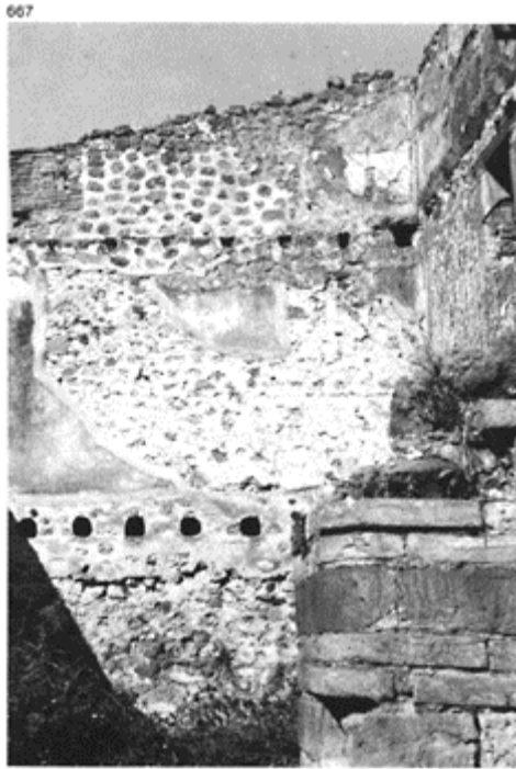
667 House of three storeys in region I, with the floor levels visible (I, 4, 28).
