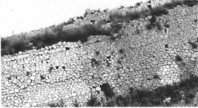
297 Walls of Terracina (between 90 and 82BC). A wall of opus caementicium , faced with opus incertum , showing the lines where the shuttering stopped.
