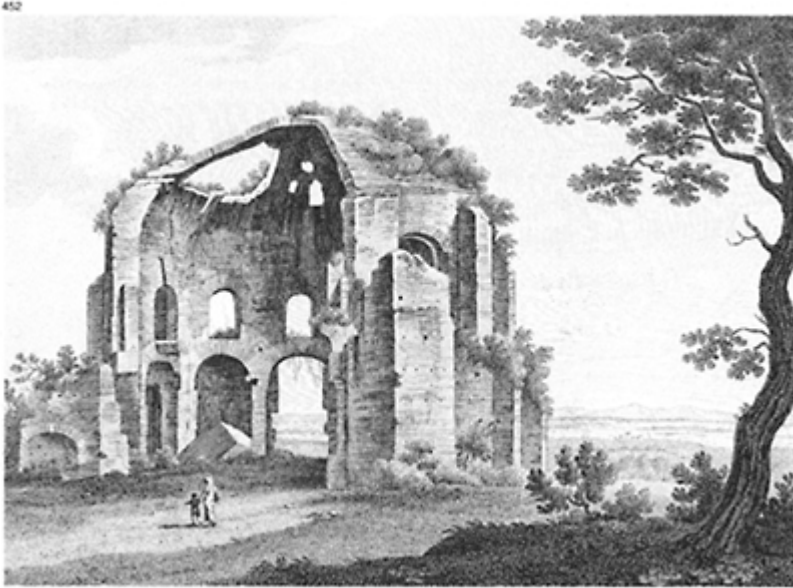
452 The dome, decagonal in plan, of the great monument of the Horti Liciniani in Rome, known as the ‘Temple of Minerva Medica’, in an engraving of 1825. At this time, the dome was still closed in. Built in the fourth century it has an internal diameter of 24.5m.
