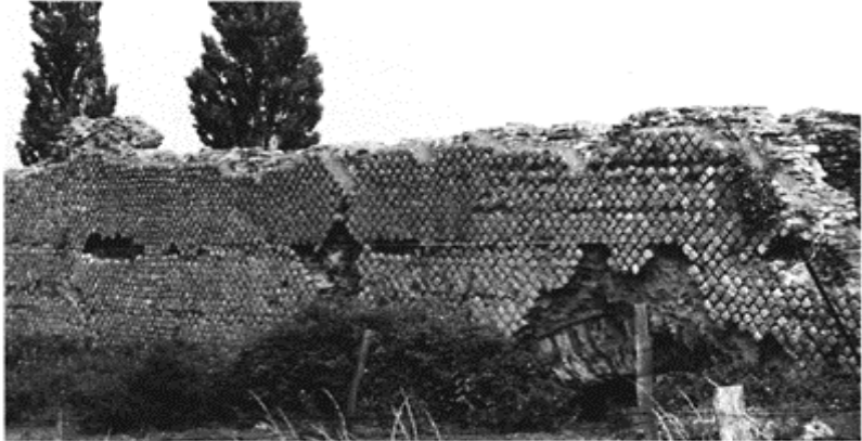
563 The aqueducts of Lyon, after crossing a depression almost parallel to the Rhône, using siphons, were for a short distance raised on sections of massive construction. The decrease in
