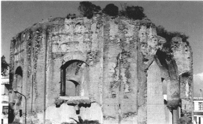
449 The 'Temple of Venus', the second great dome at the Baths of Baia, is of brick and reticulate construction; its interior diameter is 26.3m. Middle of the second century.
