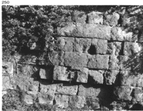
250 Ramp of the via Flaminia near the Civita Castellana. The courses of rectangular blocks of tufa follow the slope of the road with alternate rows of stretchers and rows of headers. Work began in 220BC.
