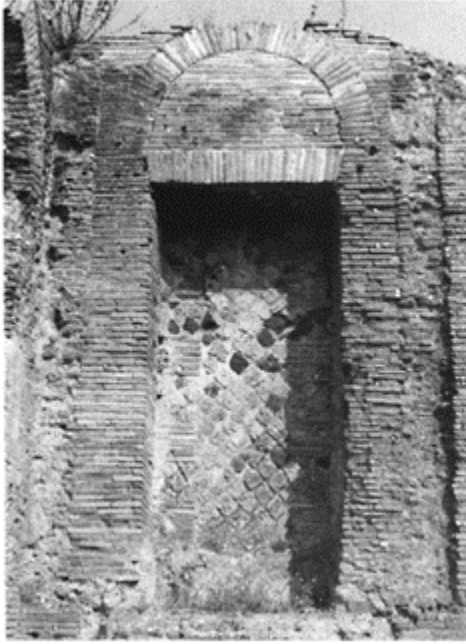
413 A bonded flat lintel without engaged voussoirs in the supports, with relieving arch. Public lararium of Pompeii, c. 60.
