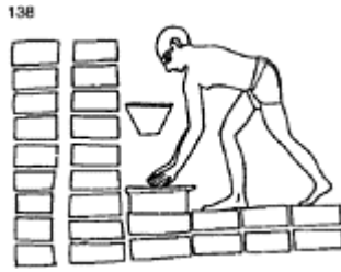
138 Moulding and drying bricks in Egypt. From a painting from the tomb of Rekhmire, Thebes (JPA).
