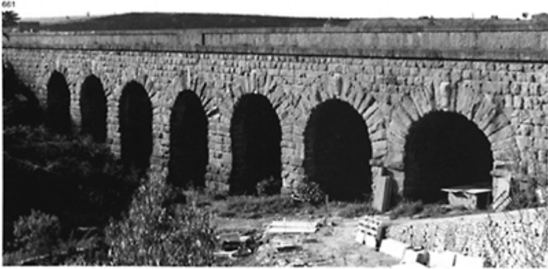
661 The Ponte di Nona on the via Praenestina at the ninth mile after leaving Rome. Length: 125m; height: 16m; c. 100BC.
