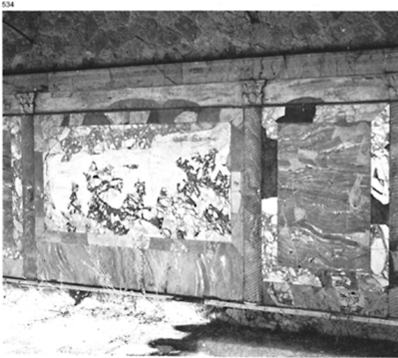
534 Wall decorated with polychrome marble panels and pilasters, in the House of the Relief of Telephus at Herculaneum, Augustan period, restored after 62.
