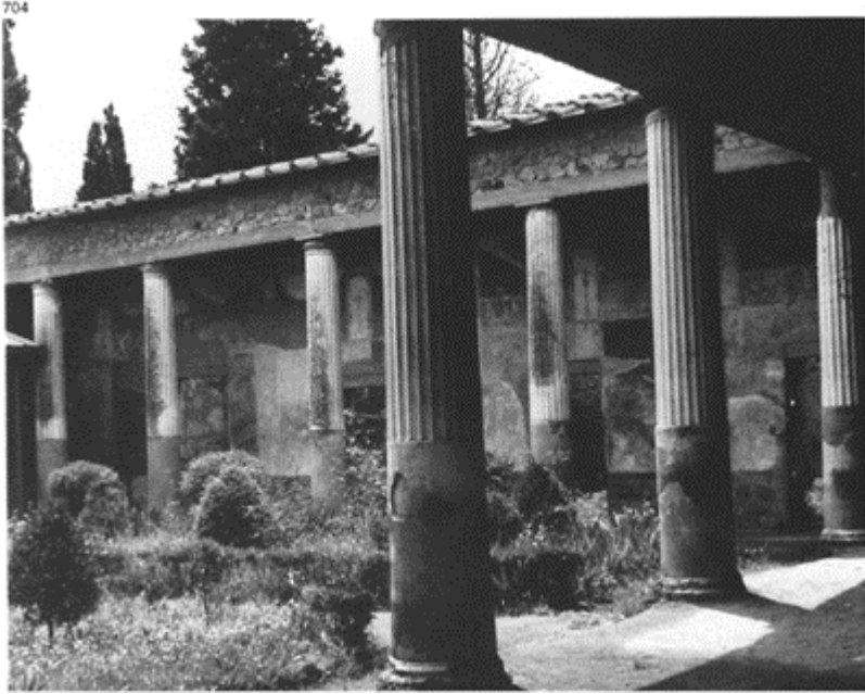
704 Peristyle in the House of Venus in the Shell (II, 3). The lowest third of the stuccoed fluted columns is protected by a covering painted red (sometimes black) in which cabling is sometimes scored.
