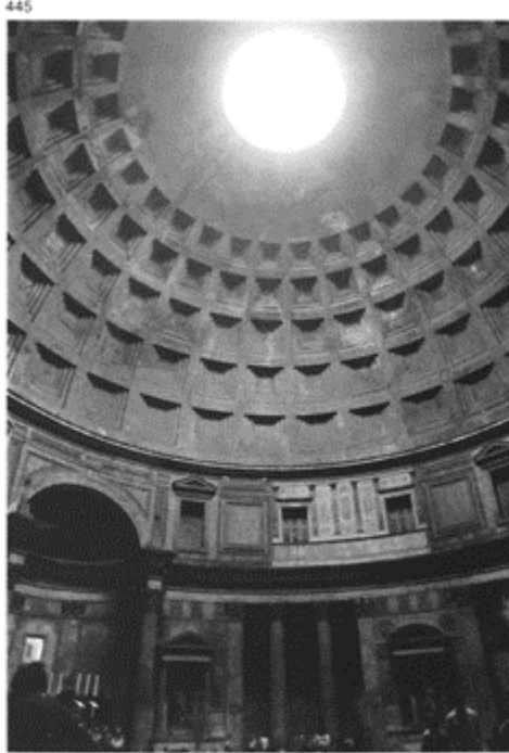
445 The unique dome of the Pantheon and its five concentric rows of coffers, lit by an oculus opening 9m across. The ancient decoration of the drum has been reconstructed in the lighter section. Diameter: 43.3m.
