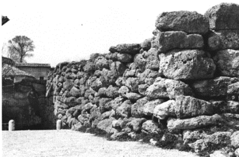
234 Walls of the acropolis of Arpino built of large stone blocks of the second type (in the background) and the first type (foreground), fifth century BC.
