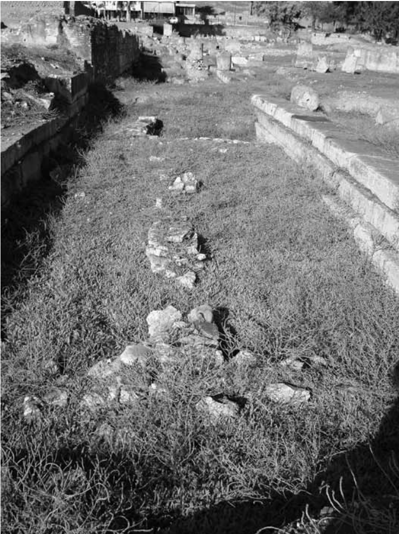
Figure 8.5: Archaic foundations beneath the northern colonnade of the southern stoa in the Argive agora from southeast (photo J.C. Donati).
