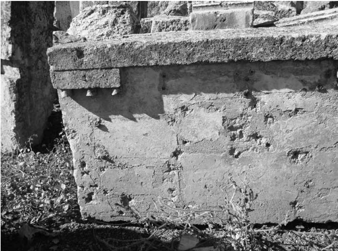
Figure 8.6: Doric architrave block with nail holes originally from the sanctuary of Apollo Lykeios in the Argive agora (photo J.C. Donati).
