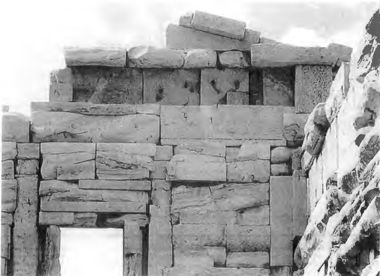
47. Erechtheion interior, west side. Statue bases in Eleusinian limestone reused in the first century B.C. as frieze background. Photo O. Palagia.
