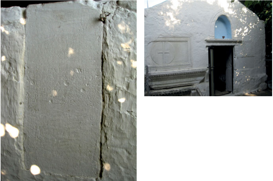
Fig. 4: The boundary stone referring to Charmylos' foundation embedded into the façade of the medieval Church of the Stavros, Pyli, Cos (photos S. Campanelli).
