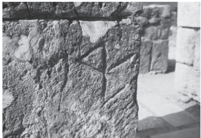
Figure 5.2 Mason's marks from Minoan palace at Malia, dated to the Late Minoan I period. Photo by author.
