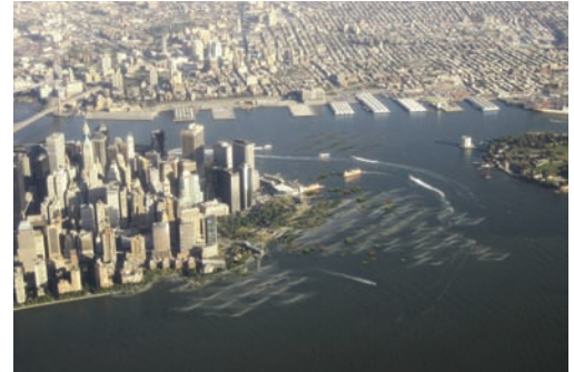
Figure 5. Lower Manhattan Zone 0 (image courtesy of Palisades Bay Team: Guy Nordenson and Associates, Catherine Seavitt Studio, Architecture Research Office).
