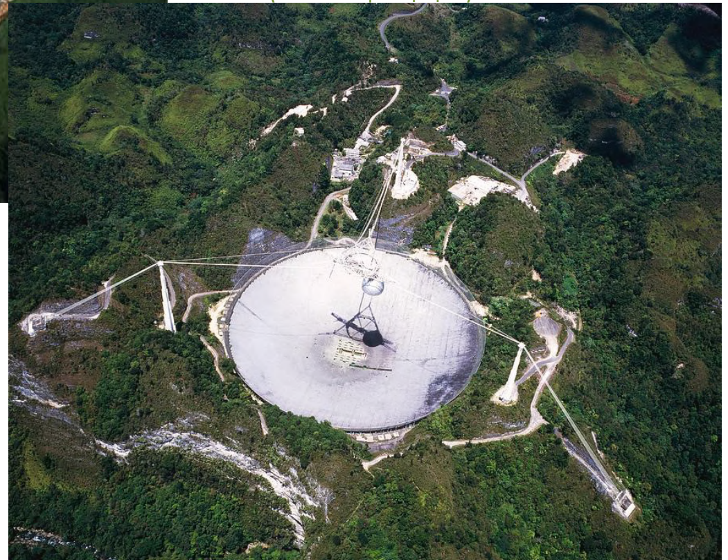
Arecibo, Puerto Rico, 300m (καταστράφηκε)
