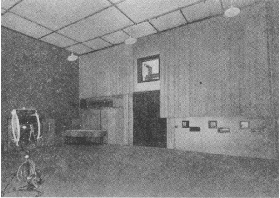
Figure 8. View of the sound stage of the Sound Motion Picture Studio of Bell Telephone Laboratories, circa 1930. The window of the monitoring booth is clearly visible. (From T. E. Shea, "A Modern Laboratory for the Study of Sound Picture Problems," Journal of the Society of Motion Picture Engineers , March 1931, page 278.)
