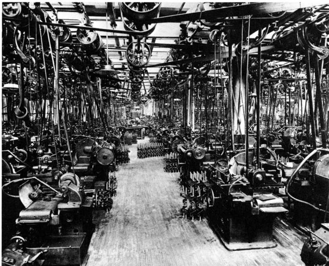
FIGURE 6.8. Ford Crankshaft Grinding Machines, 1915. Developments in grinding technology, such as the machinery for grinding crankshafts, played an important part in the achievement of accurately machined automobile parts. (Henry Ford Museum, The Edison Institute. Neg. No. 833-2296.)
