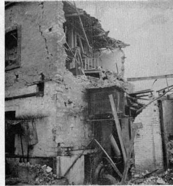
Fig. 5: A picture of damage done to houses of a very poor construction in Pharsala, Thessalia, during the earthquake of March 8, 1957.
