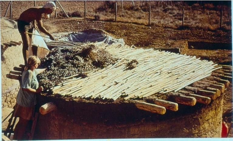
28. The roof of Roundhouse 3 rests on rafters laid across the wall head and covered with layers of bam-
