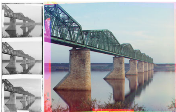
Fig. 2.73 Sergei Gorskii, Trans-Siberian Railway metal truss bridge on stone piers, over the Kama River near Perm, Ural Mountains Region, c.1910
