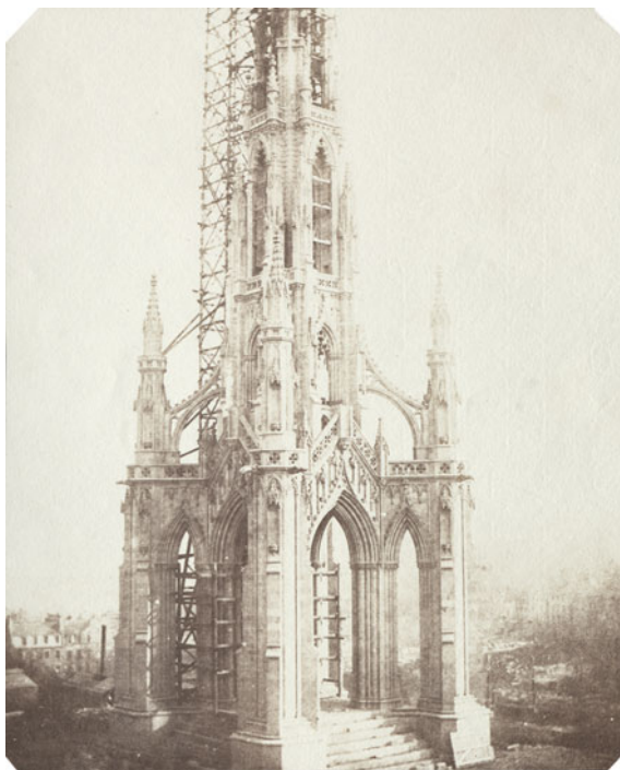
Fig. 2.28 Sun Pictures in Scotland: Scott Monument Under Construction. The Cleveland Museum of Art, Andrew R. and Martha Holden Jennings Fund 1987.23
