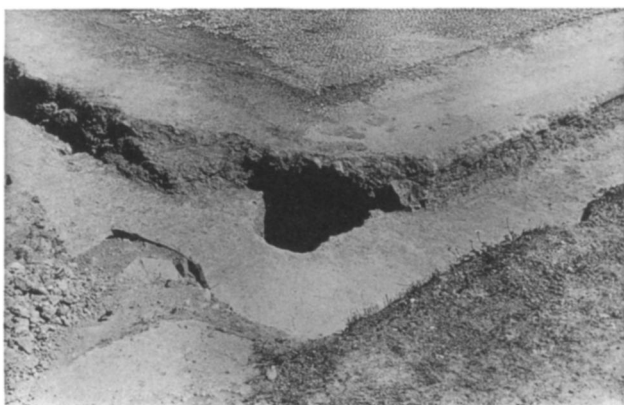
3. Manhole under Square
