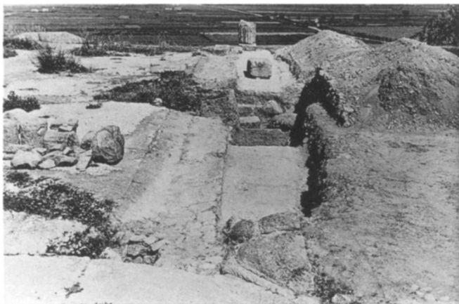
1. East Stylobate Foundations
