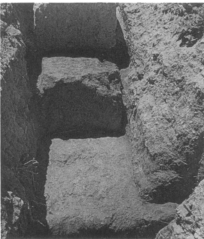
5. Brick Core against a Tie-Wall
