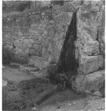
2. Exterior Facing at End of Drain Channels
