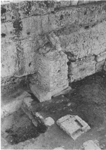
1. Ramp Gate Center Block
