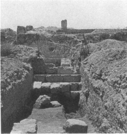
1. Exterior Facing Foundations
