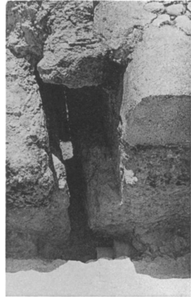
3. Rock-Cut Channel H to Shaft S
