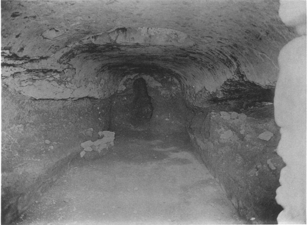
1. Reservoir II, Interior
