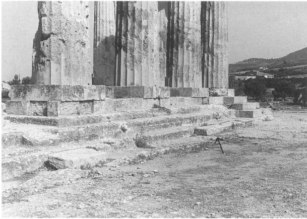
FIGURE 7.26. Temple of Apollo, west facade (arrow points to euthynteria blocks with claw chisel marks)
