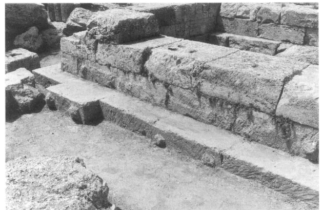
FIGURE 7.13. Temple of Hera Akraia at Perachora, foundations of the south wall
