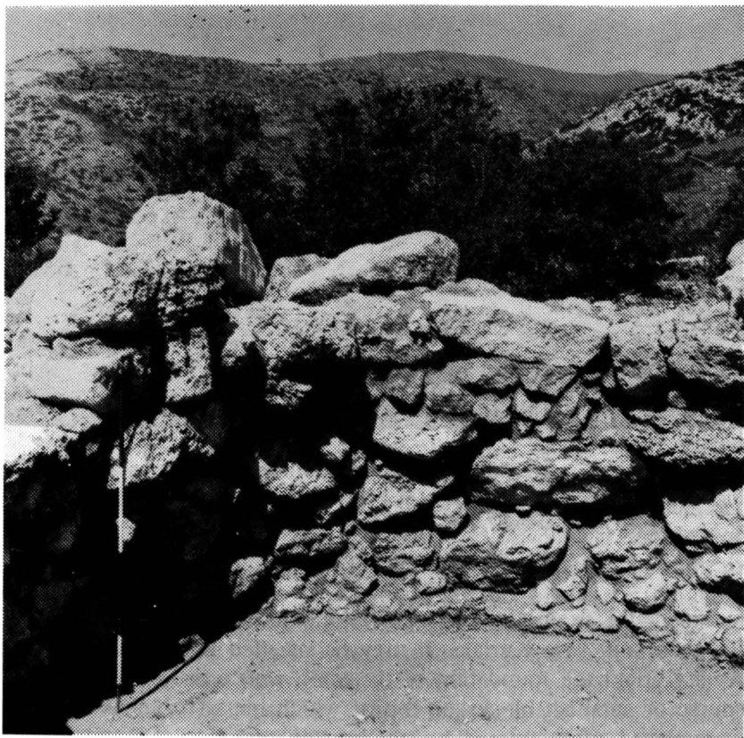
Figure 3.6 Part of the wall of Megaloi Skinoi A, preserved to a maximum height of 3.4m (the author).
