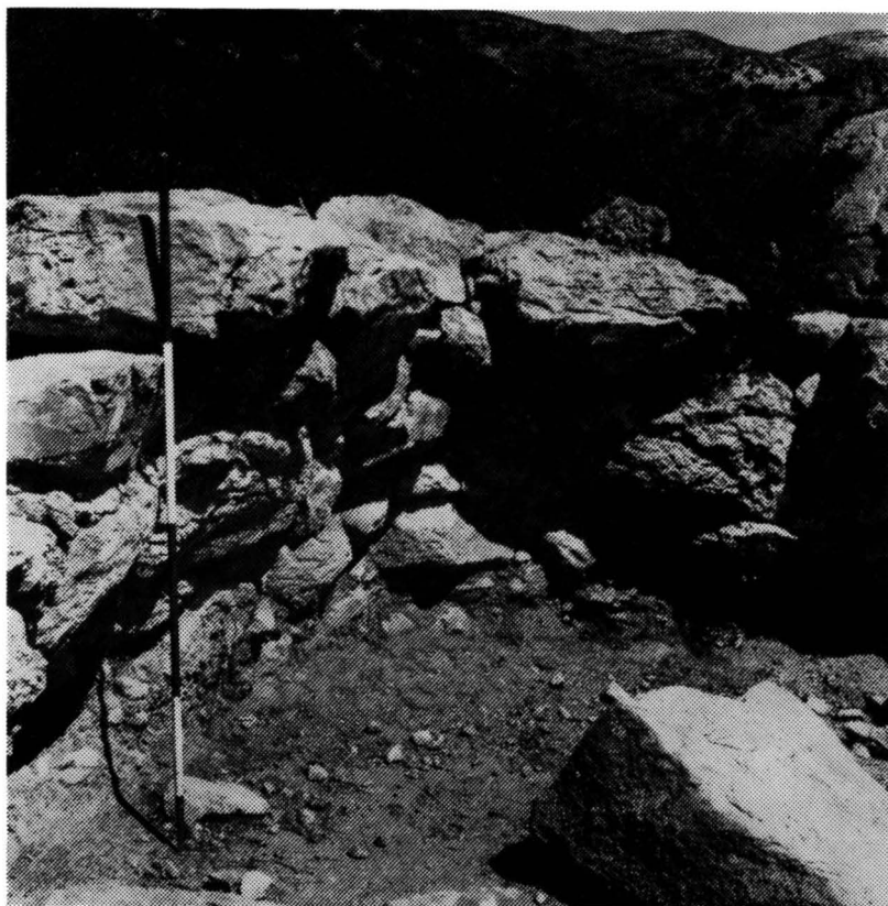
Figure 2.3 Corbelling and the resulting overhang on the north side of the tomb wall at Ayia Kyriaki (the author).
